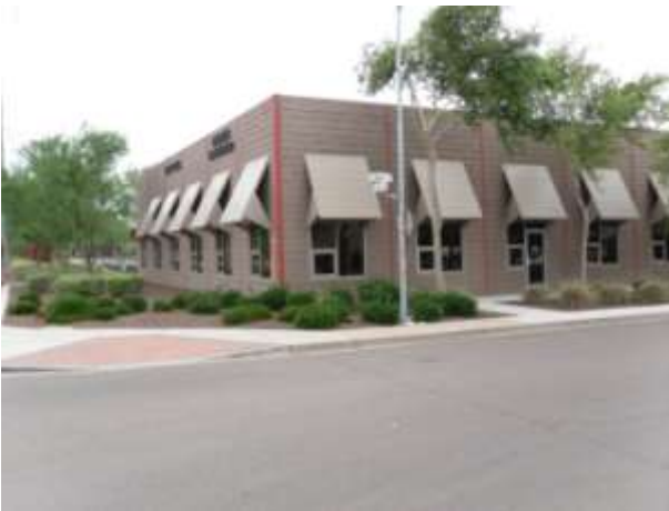
Rear/Side View Of Subject Unit
